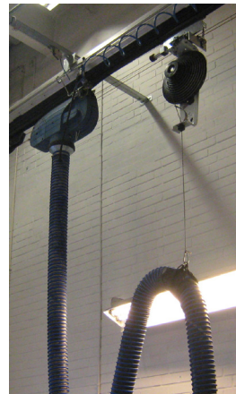
Suction unit 920/1500 together with extra balancer trolley and 831 Balancer
